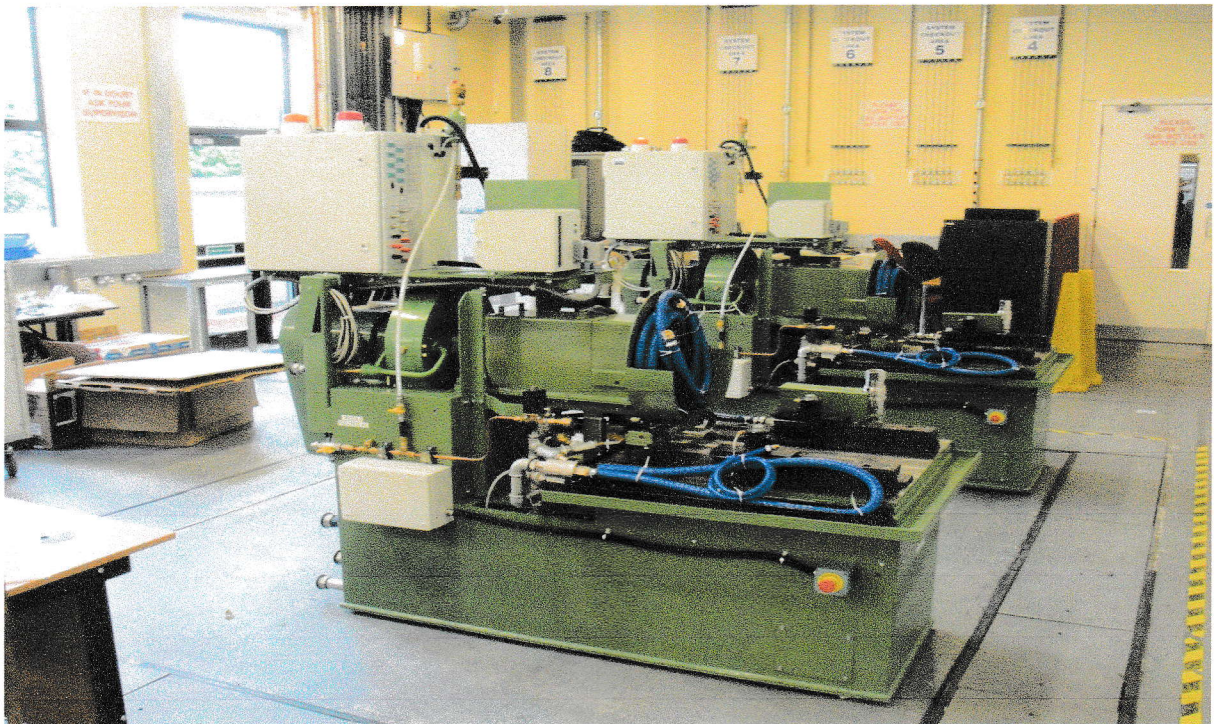
Perkins Shibaura engine test beds for Wuxi China during build and installation at Griifin USA
