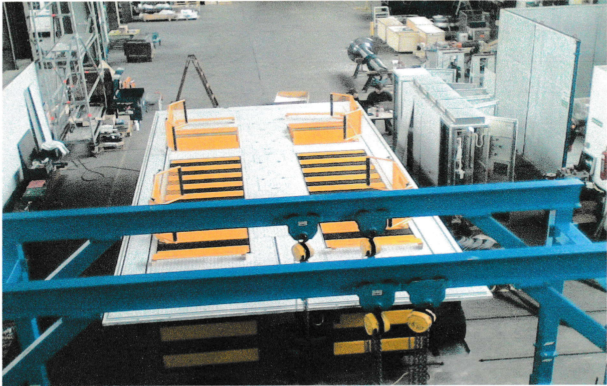
Shop-build of a 48" Chassis Dynamometer for VW Wolfsburg.
