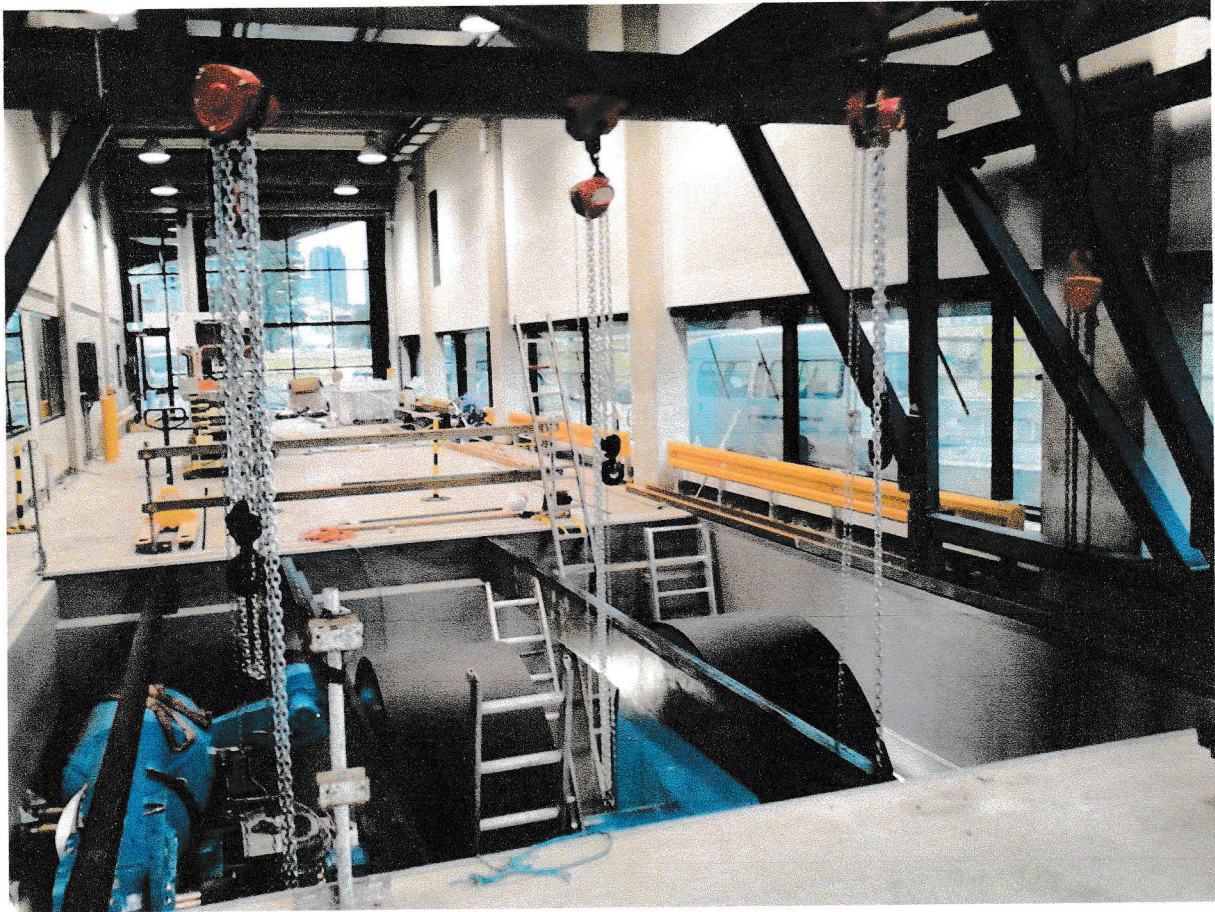
Our 16,000kg SWL lifting gantry during the installation at Kangan Institute, Melbourne, Australia.
